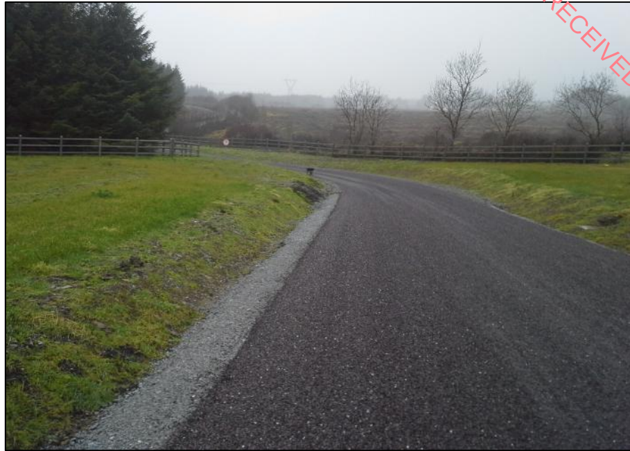
Figure 5-6 - Completed Access Track
