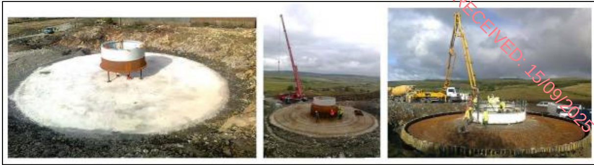
Figure 5-9 - Turbine Foundation Formation, Steel Reinforcement and Concrete Pour
