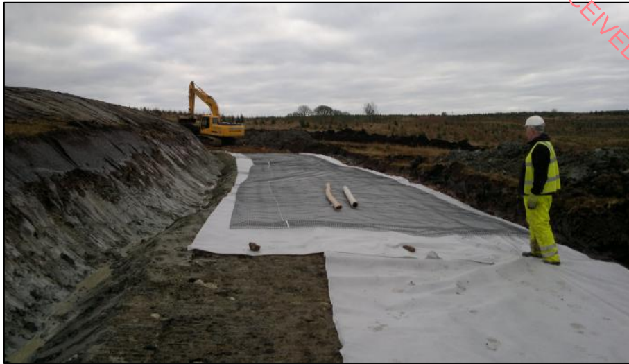
Figure 5-5 - Excavated Access Track Formation, Geotextile, Geogrid and Edge Drain
