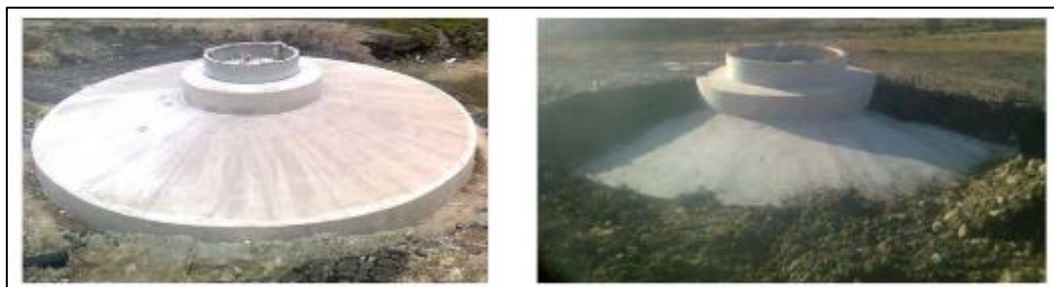
Figure 5-11 - Wind Turbine Foundation Backfilling
