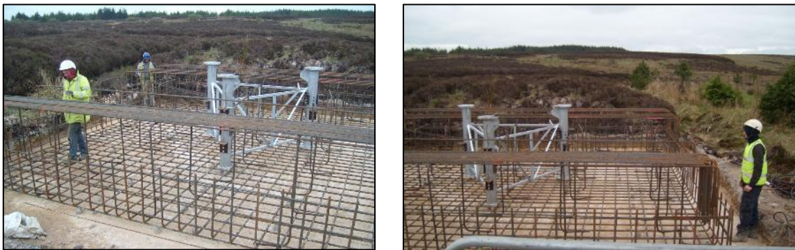
Figure 5-14 – Communications Relay Tower Base Construction
