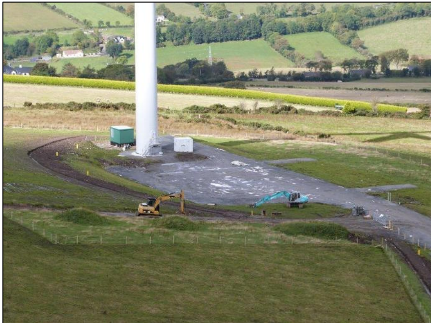
Figure 5-15 - Turbine Foundation and Hardstand Reinstatement
