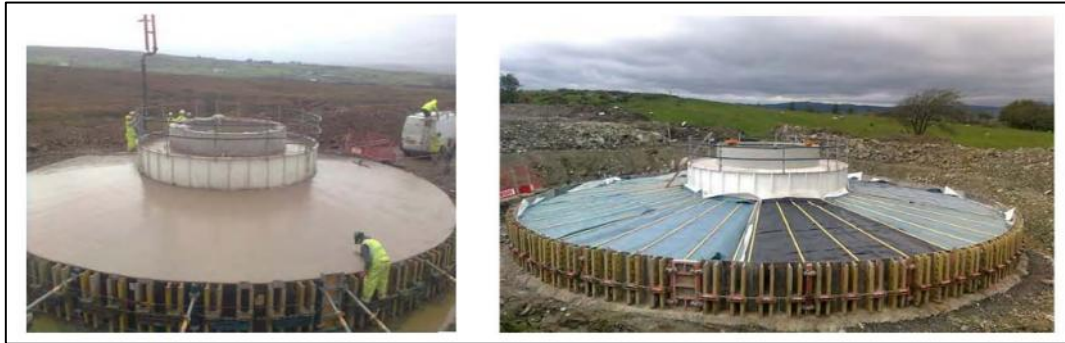
Figure 5-10 - Wind Turbine Shuttering, Finishing and Curing
