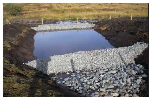
Figure 5-3 - Settlement Pond Construction in advance of the Works, and later its operation
