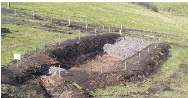
Figure 5-3 - Settlement Pond Construction in advance of the Works, and later its operation
