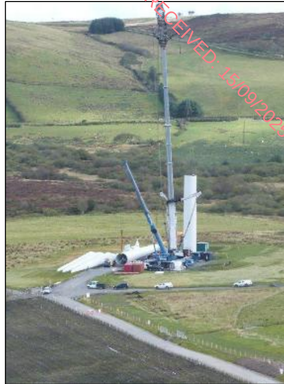
Figure 5-12 - Wind Turbine Erection
